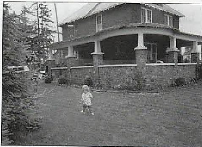
The Sutherland house on Lot 2, Concession 1. It took Clifford Sutherland and his son Stanley about five years to build the wrap-around veranda, using stones gathered on their fields and the fields of their neighbours. Playing on the lawn are current residents Sonya (left) and Lesley Sutherland.
